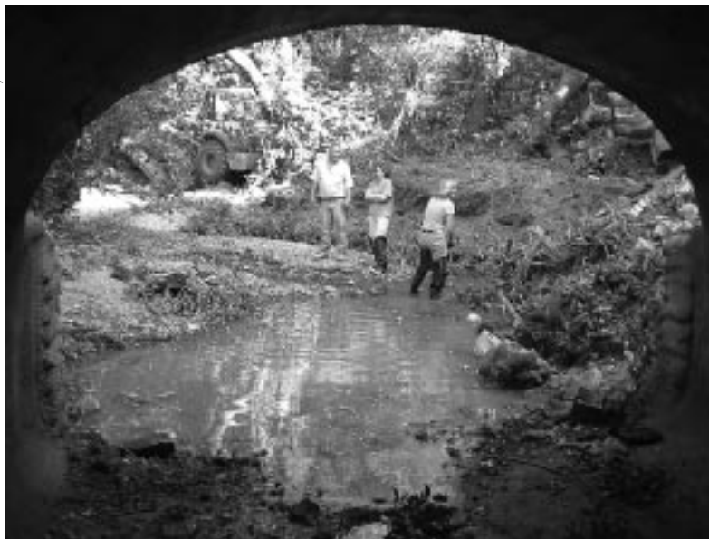
L to R: James Reagan Jr., Kallie Kull, and Liz Lewis make a final assessment of the culvert to be removed in the salmon restoration project.
