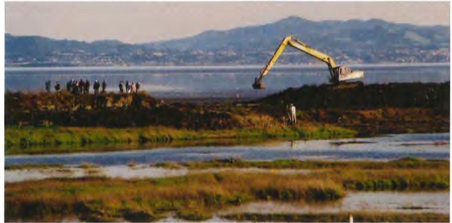
A levee is breached at Tubbs Island, allowing the Bay’s tides to come in and recreate tidal marsh. Photo by Marc Holmes.
