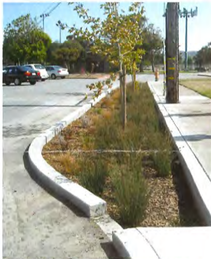
A curb extension in San Bruno (notice the cut in the curb). Photo courtesy San Mateo County.
