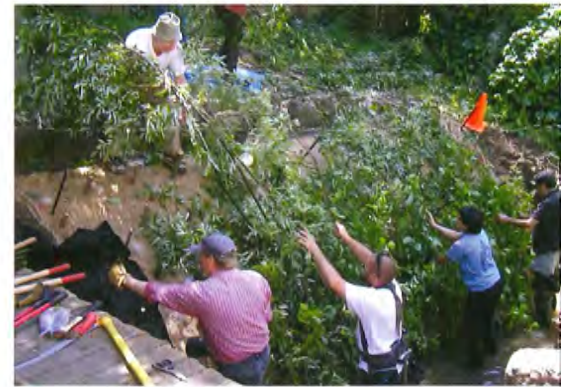
"Soil bioengineering" is a way to stabilize and green creek banks using plant material instead of riprap. It helps make our watersheds more resilient. Photo courtesy of Urban Creeks Council.
