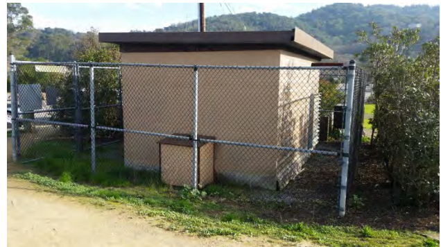
Stormwater Pump Station in Santa Venetia. Credit: BVB Consulting LLC
