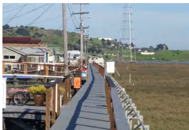
Greenbrae Boardwalk. Credit: BYB Consulting LLC
