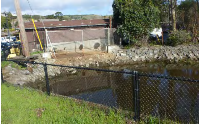
Pump station and overflow pond at the Cove Shopping Center. Credit: Marin County DPW
