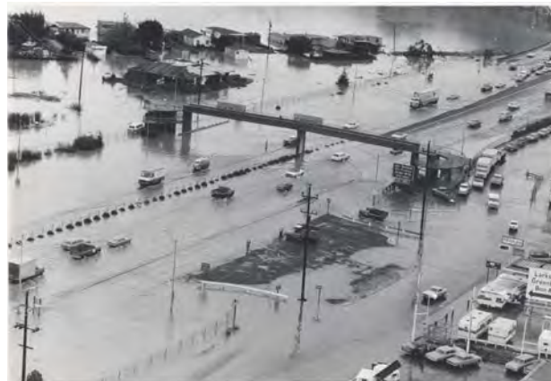
1973 Flood on US Highway 101 and fronting marshes. Larkspur. Credit: Marin County DPW
