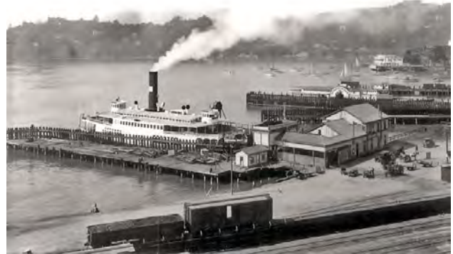
Tiburon once served as the southern terminus of the Northwestern Pacific Railroad. Credit: Photographer on San Francisco and North Pacific Railroad Station House-Depot National Register of Historic Places Nomination Form
