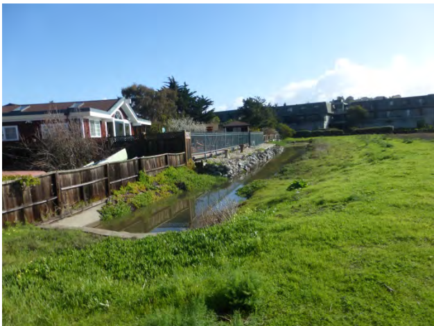
Vulnerable homes bordering Greenwood Cove. Feb. 18, 2016. Credit: Marin County DPW.
