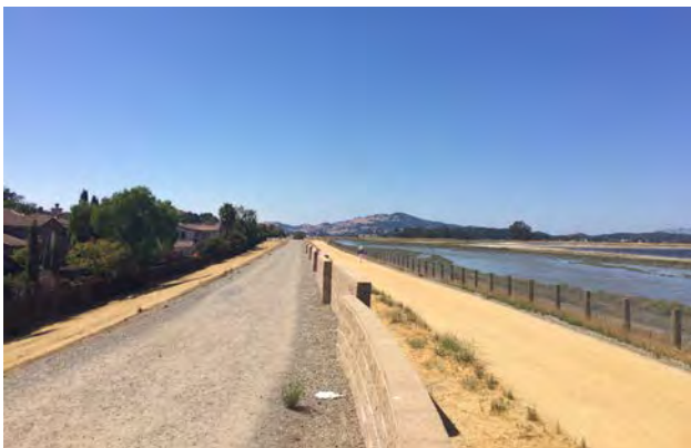
Hamilton levee and pathway. Credit: Marin County CDA
