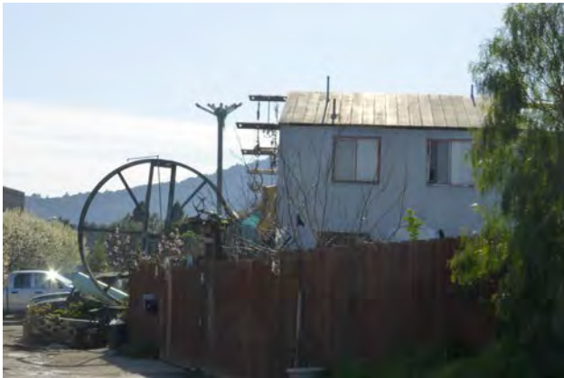
Housing at the end of Lucky Drive. Corte Madera. Credit: Marin County DPW
