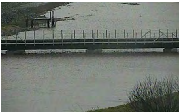
SMART Bridge, Novato. Credit: Marin County DPW
