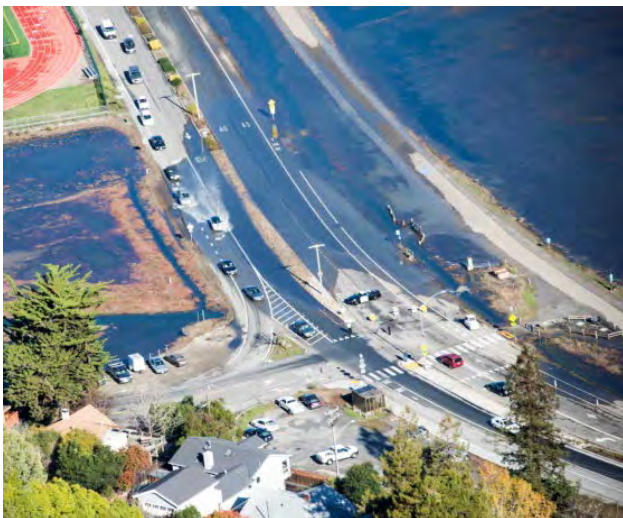
King tides preview future water levels. Mill Valley. 10:41 a.m., Nov. 25, 2015. Credit: Light Hawk Aerial
