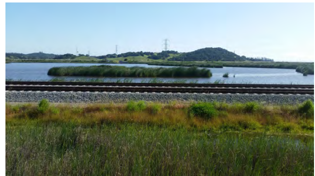
SMART railroad in Novato. Credit: BVB Consulting LLC
