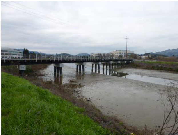
SMART Rail Bridge, Novato. Credit: Marin County DPW
