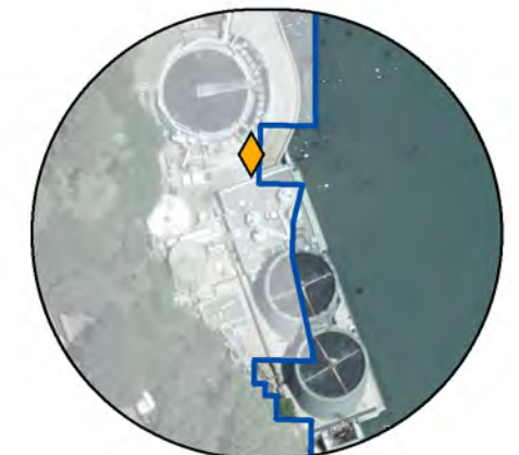
4: Sausalito Marin City Wastewater Treatment Plant
