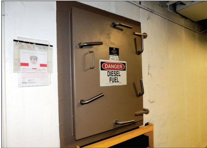
Flood-proofed generator door
