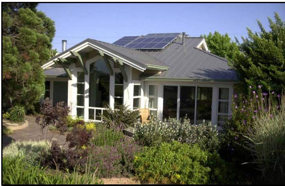
Figure E-1 Residence with Solar Photovoltaic Energy System
