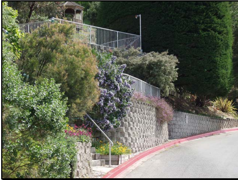
Figure C-8 Inappropriate Retaining Wall Design
