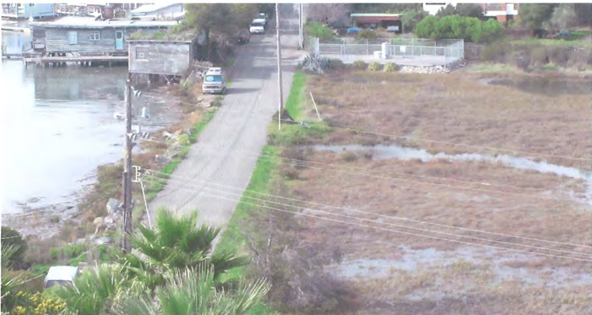
A 24 inch culvert chokes the 5 acre Beach Drive Marsh promoting Spartina growth
