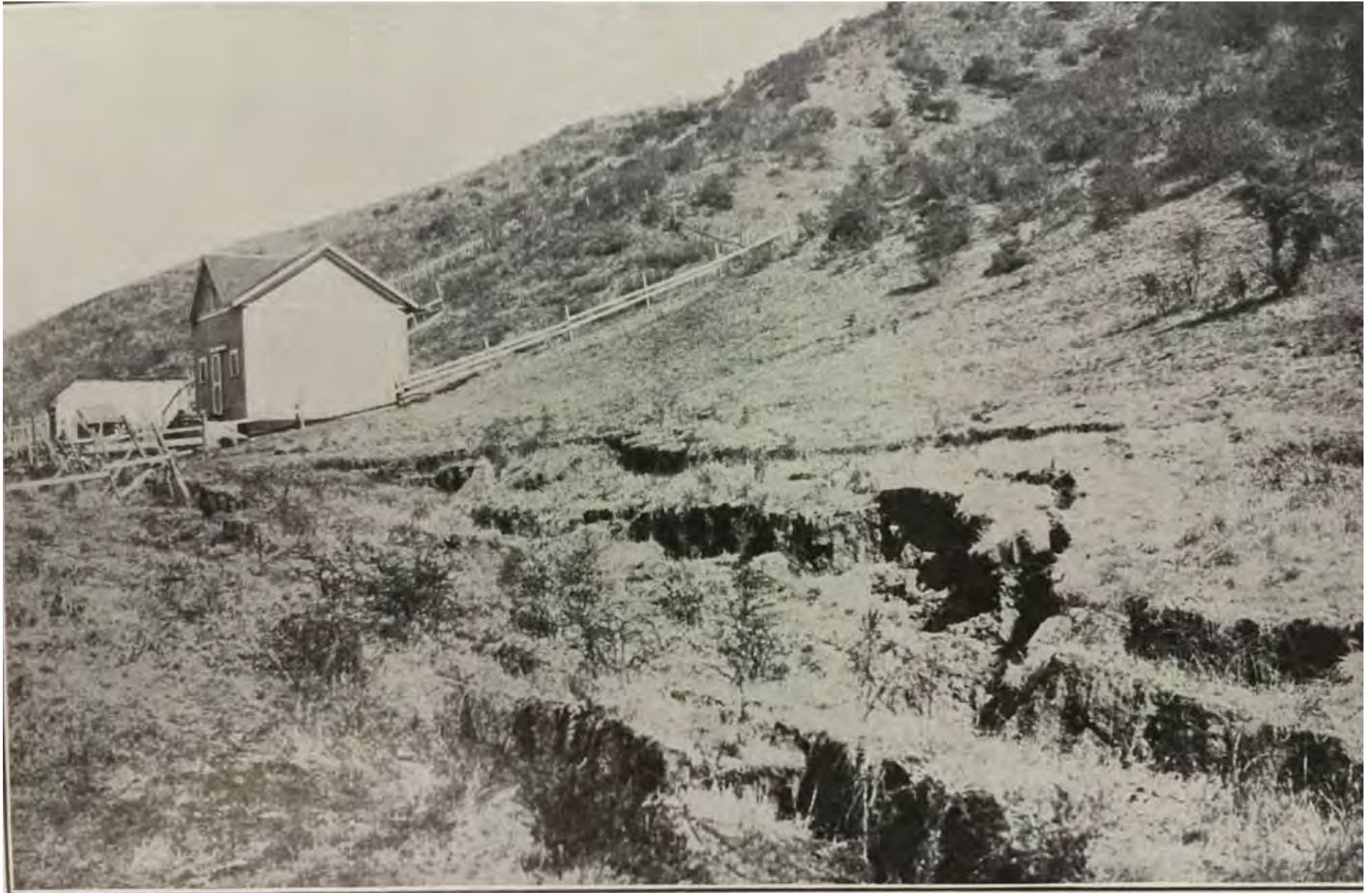
Secondary cracks with settling, Bolinas. Photographed by G.K. Gilbert. From: San Francisco Earthquake and Fire of April 18, 1906 and their effects of structures and structural materials, reports by Karl Gilbert, Richard Lewis Humphrey, John Stephen Sewell, and Frank Soule, Washington Government Printing Office, 1907.
