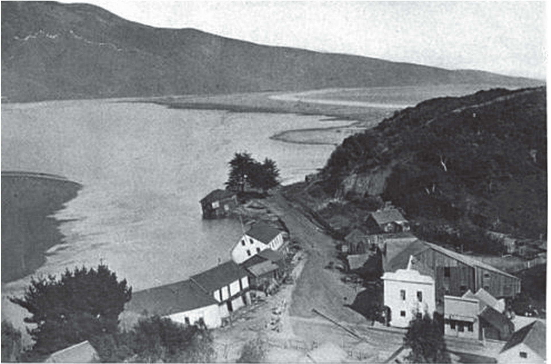
Looking down Bolinas Bay and Lagoon toward Golden Gate. Village of Bolinas in foreground. H.W.F. The California Earthquake of April 8, 1906: Report of the State Earthquake Commission by California Earthquake Investigation Commission, by Andrew Cowper Lawson, published by the Carnegie Institution of Washington, April 1908, V1.
