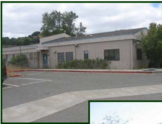
Future site of the Juvenile Hall sally port. Photo taken on May 30, 2008.
