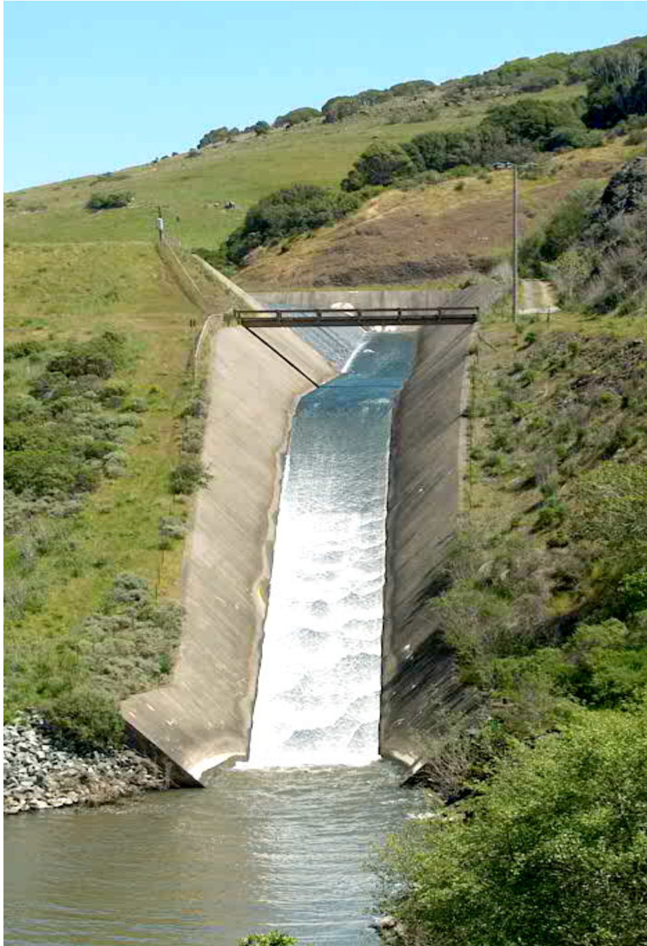
Lake Nicasio Spillway April 18, 2005
