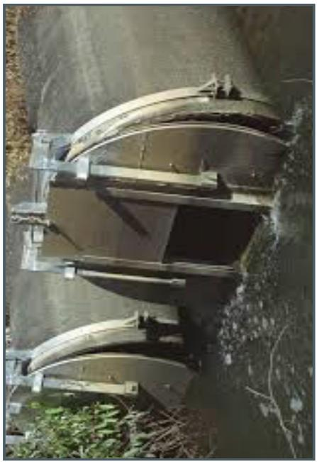
Tide gates can be used in conjunction with pump stations to increase water circulation
