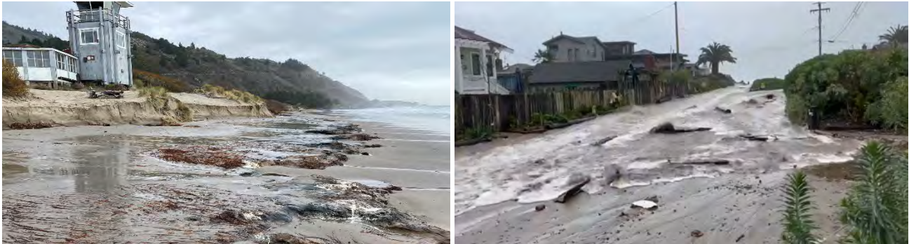
January 5, 2023 coastal storm impacts at Stinson Beach: (left) beach and dune erosion at NPS Lifeguard Station (Source: Twitter @WestMarinFeed) and (right) wave overtopping on Calle del Resaca Twitter @Sammy_Herdman).
