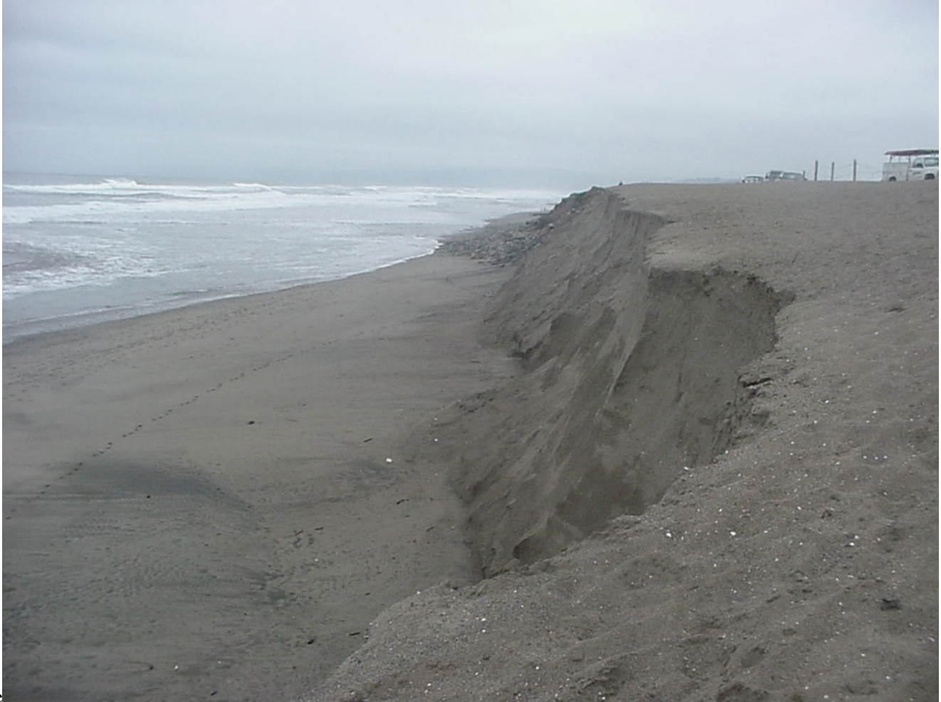
Figure 16 Scarp at eroded dune embankment, Ocean Beach, San Francisco
