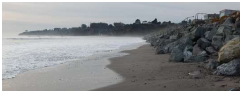
Example of reduced lateral access along Seadrift rock revetment in winter illustrates potential long term beach conditions with sea-level rise and/or post-storm conditions for the traditional armoring baseline (Peter Baye 2019)
