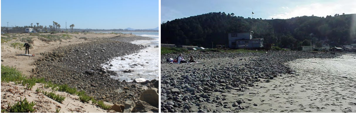
Sand lens atop constructed cobble berms at Surfer’s Beach in Ventura County (left) and Pacifica State Beach (right). Source: Bob Battalio
