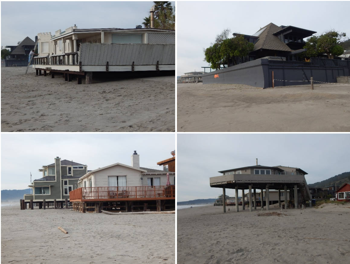
Calles reach, December 20, 2019. Homes are located on the active foreshore and backshore (swash zones of fair-weather and storm beach profiles); eroded foredunes, where they persist, are landward and between the prominent homes. (P. Baye)
