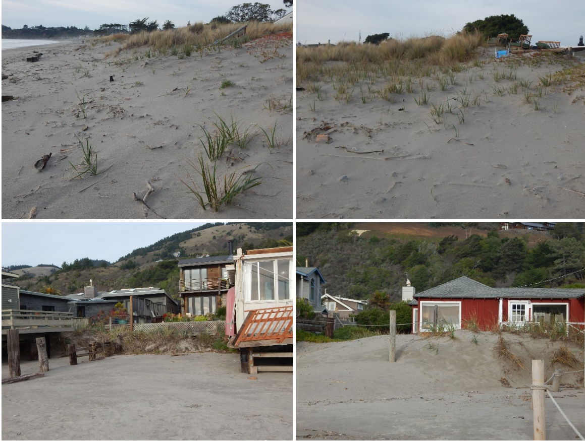
Beach wildrye was apparently planted on sand embankments placed in front of set-back residences within the Calles reach. The sand embankments and wildrye are mostly eroding by undercutting from wave action. (P. Baye)
