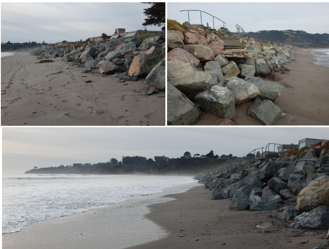
Western rock revetment in Seadrift reach, December 20, 2019. Intertidal beach face is revealed at low tide, the surf zone reaches the revetment at high tide with no backshore. An apparent foreshore trough with visible longshore currents lies close inshore near the beach face. (P. Baye)
