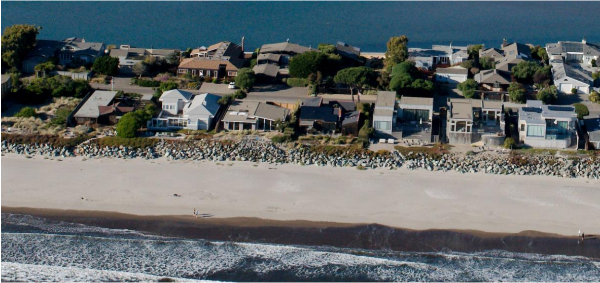
Figure 8. Existing rock revetment fronting Seadrift homes. Source: californiacoastline.org (2013).
