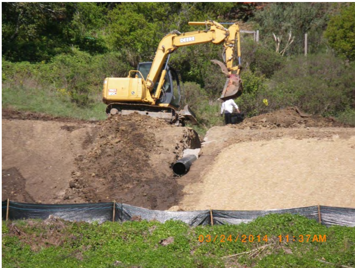
Figure 10. Culvert Installation on 3/24/2014 - Size and proper installation BMPs unknown. Source of fill dirt unknown. AR 00950
