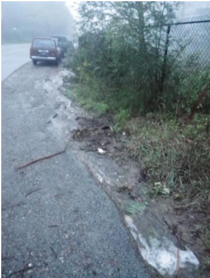
Downcutting of diverted water on Panoramic shoulder reaching creek eventually further down.
