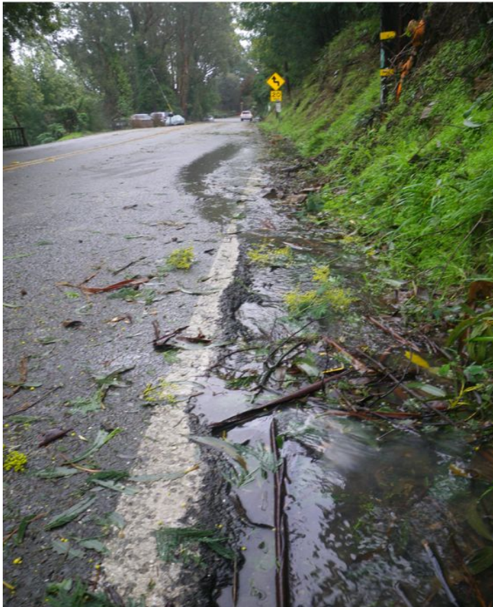
Clogged inboard ditch that floods our property and where road entrance is going to be added. January 17, 2019
