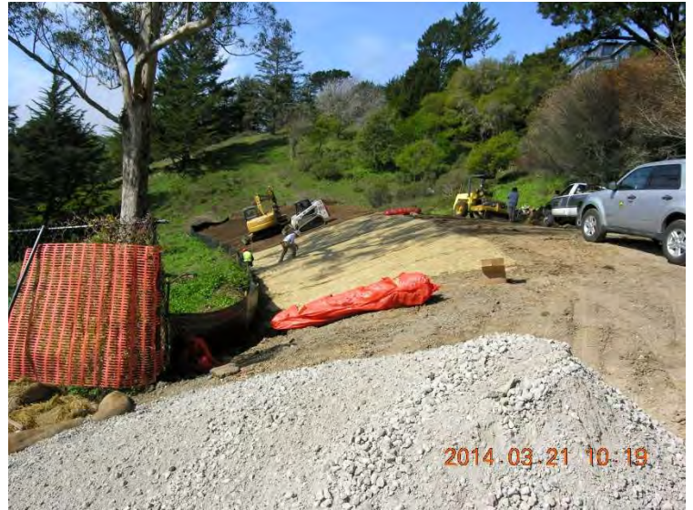
Photograph 2. Grading activities under way, March 2014
