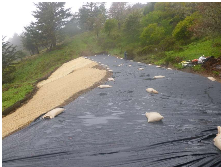
Photograph 3. Grading complete, BMPs installed. March 2014
