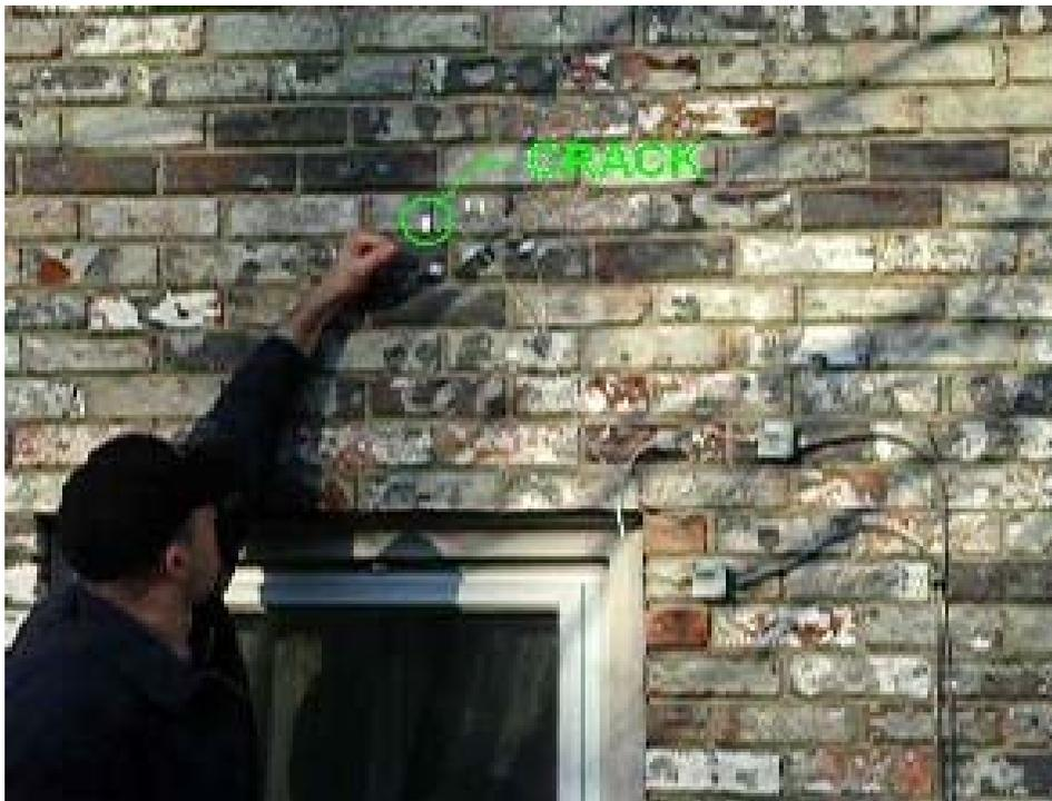
Figure 2.9 – Crack Gauge Installed over a Crack in an Exterior Brick Wall
