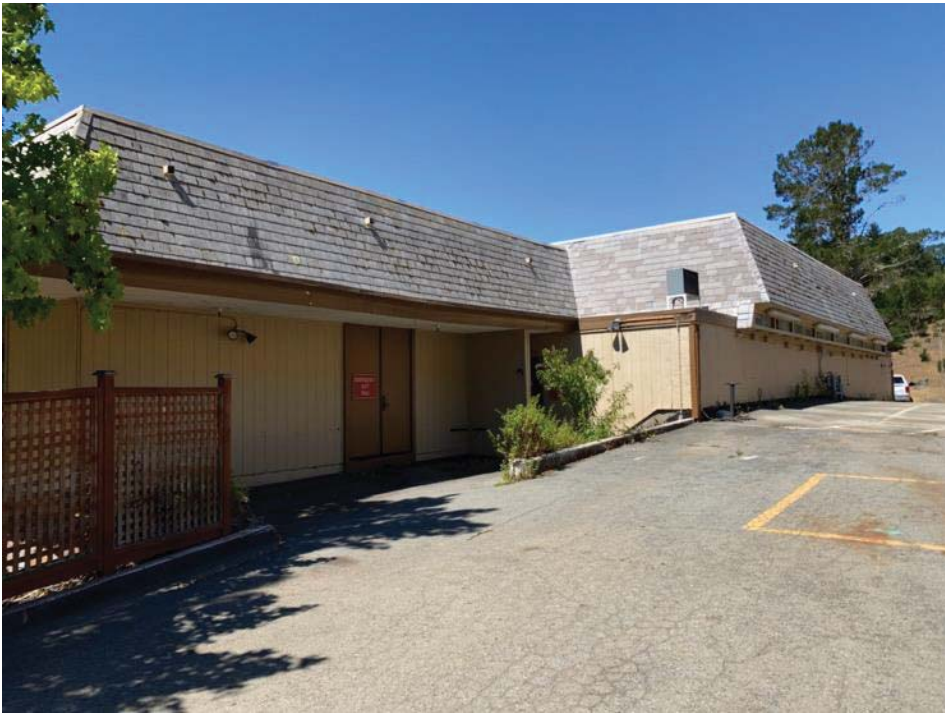
Figure 10. Partial north elevation showing rear fire exit, view looking southwest
