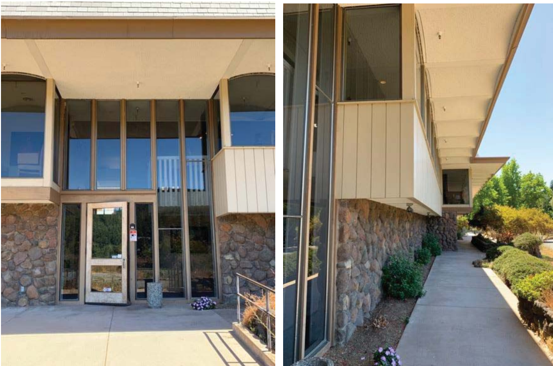
Figure 4- 5. Detail views of primary entry on south elevation (left) and roof eave and overhang (right)
