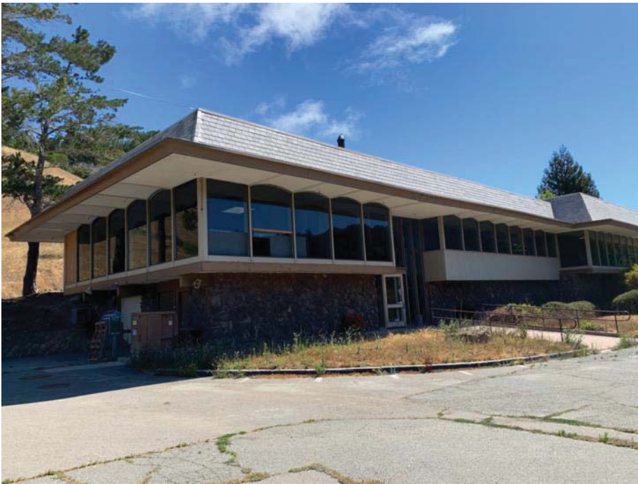
Figure 2. South and west elevations, view looking northeast
