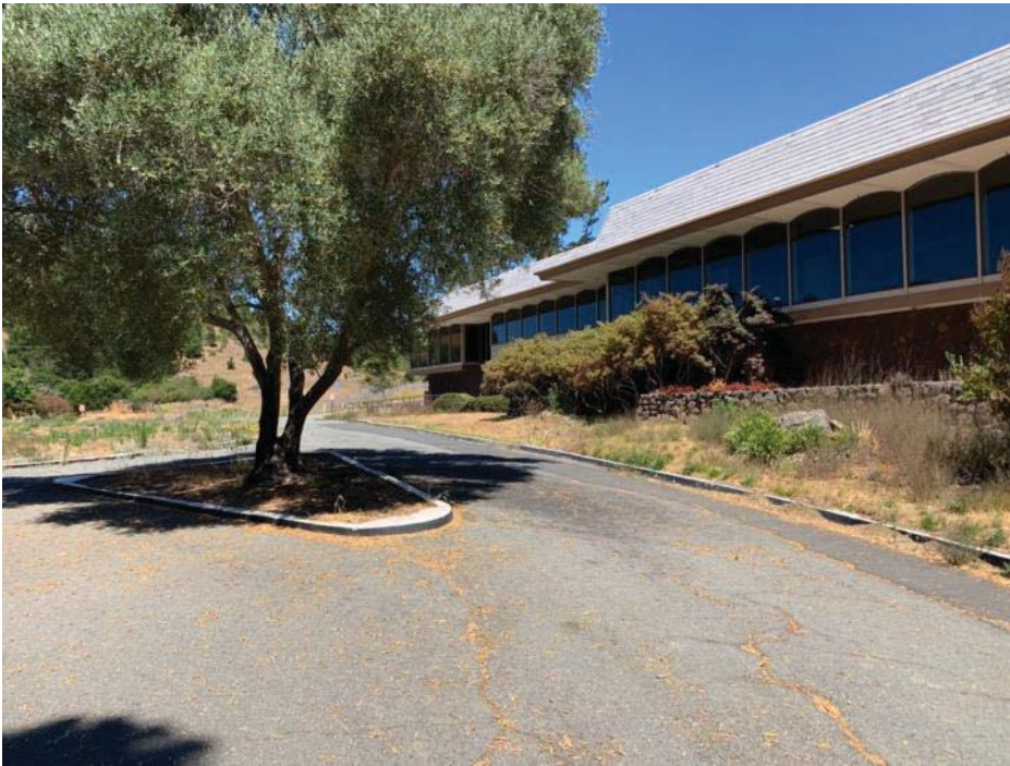
Figure 18. Circular driveway at club house entrance, view looking northwest
