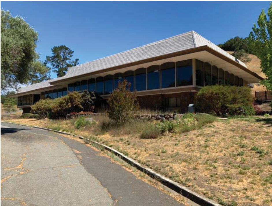
Figure 1. South and east elevations, view looking northwest
