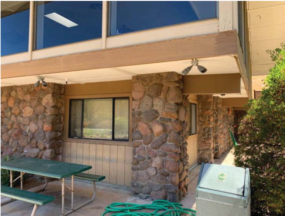
Figure 6. Detail view of southeast corner, ground floor, view looking northwest
