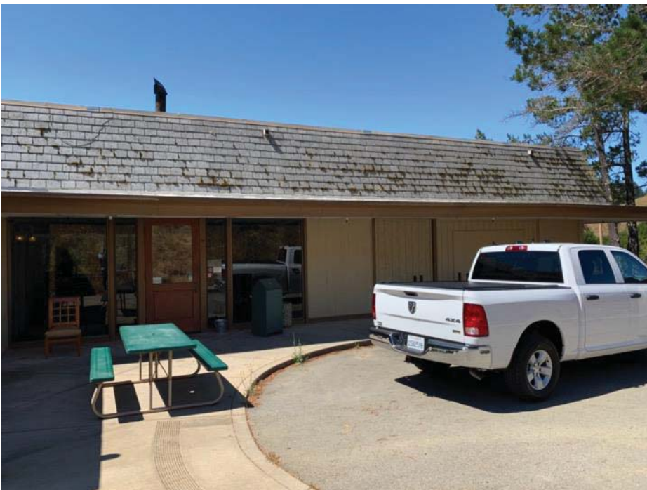
Figure 9. Partial north elevation showing rear entrance, view looking south
