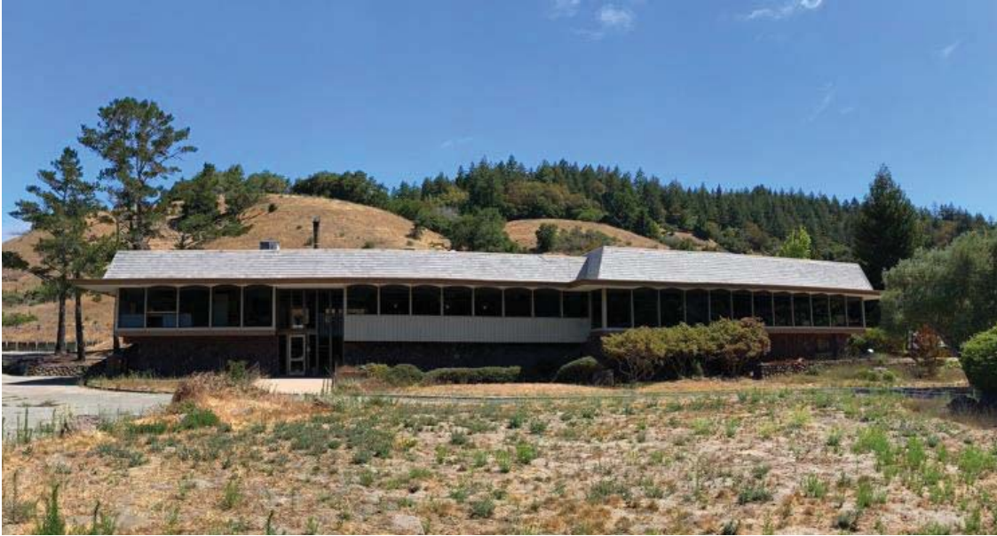
Figure 3. Panoramic view of south elevation, view looking north
