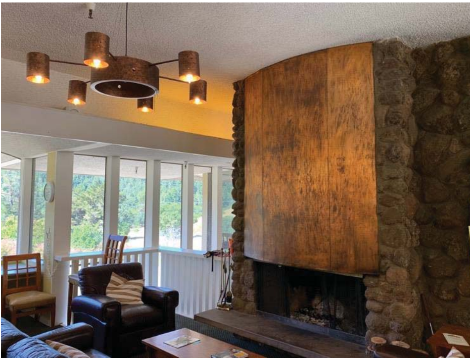
Figure 11. Lava rock and copper clad fireplace in bar/lounge area, view looking southwest
