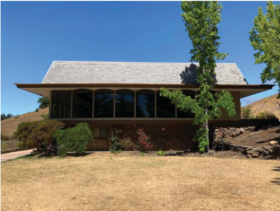
Figure 7. East elevation, view looking west
