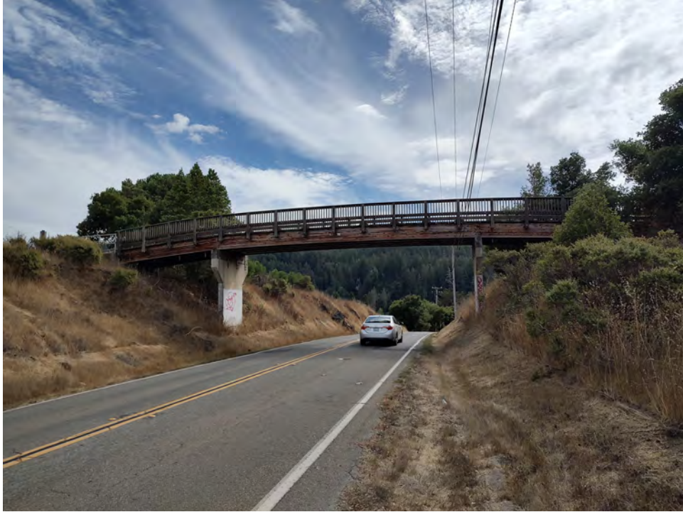
Figure IV.1-3: Bridge over Nicasio Valley Road
