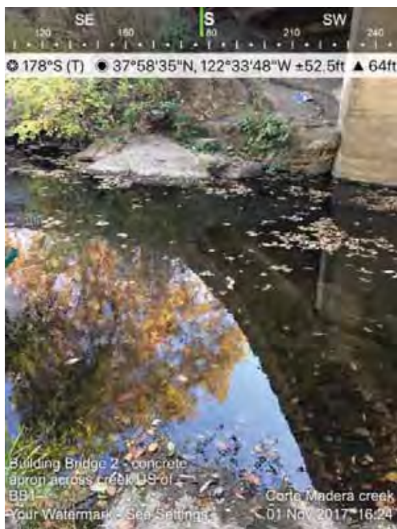
Figure A-16: Concrete Sill Extending across Channel on Downstream Face of Bridge Street Bridge
