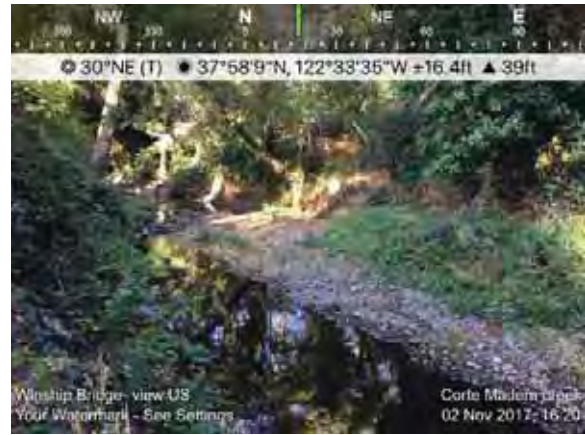
Figure A-19: Looking Upstream at Channel Upstream of Winship Avenue Bridge
