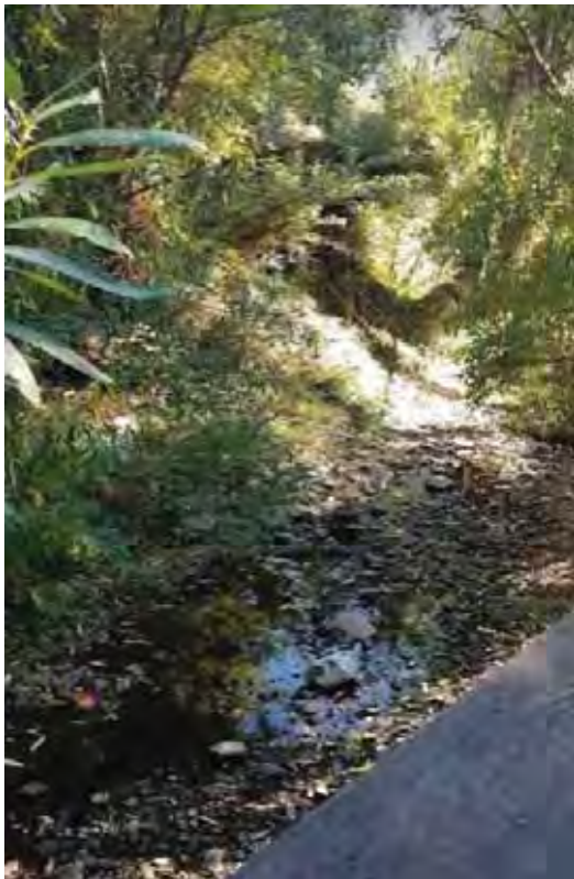
Figure A-5: Azalea Avenue Bridge Upstream View
