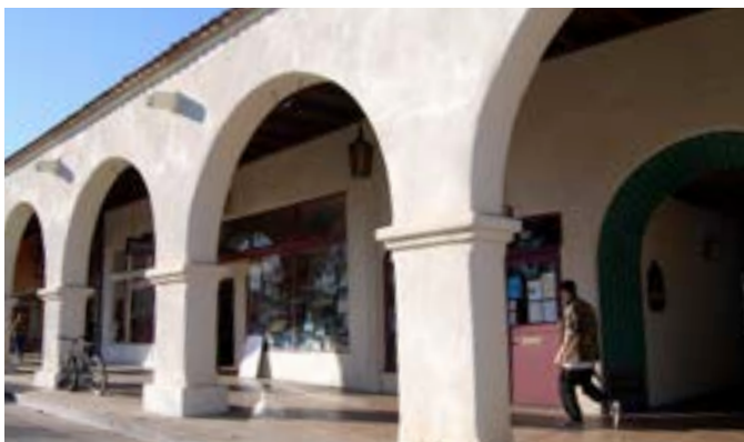
Example of a Gallery with shopfronts
