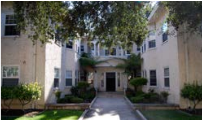
Example of Forecourt
