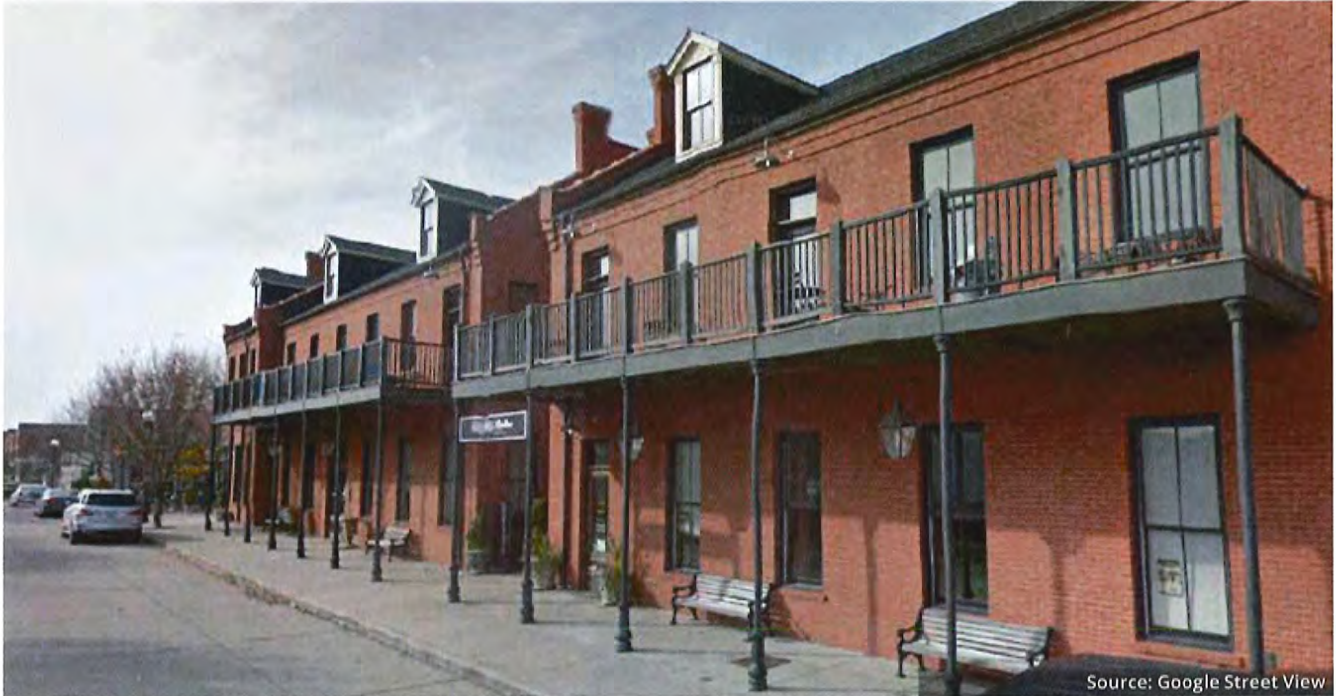
Example of a two-story Gallery with an uncovered second story.
