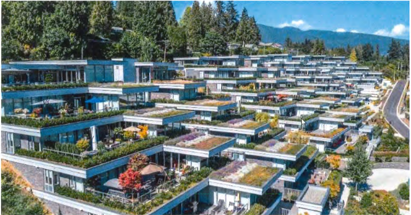
Example of Terraced Courtyard Building (Courtesy of ONNI)
