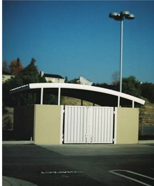
Figure 3.1. Roofed and bermed refuse area.
