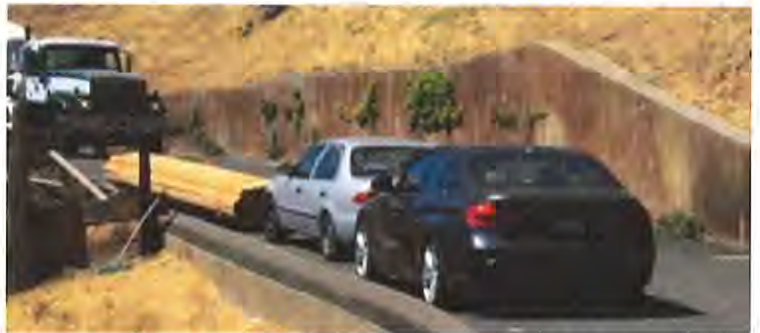
Retaining wall along Sacramento Ave with attempted vegetation screening (and blocked fire access).
