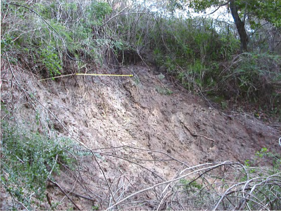
Fig. 2. Top portion of slide, below steep hillside development site. Measuring tape = 10 feet.
