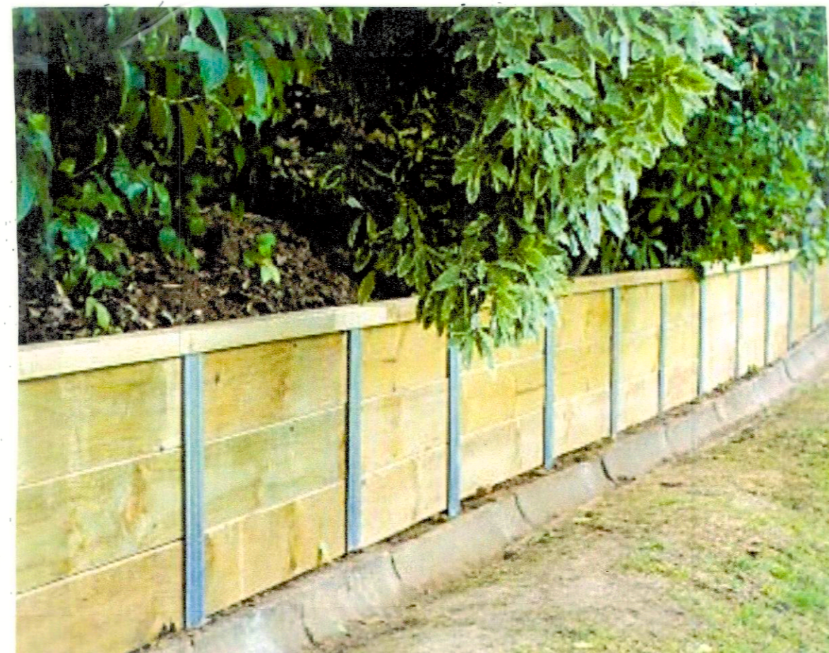
TYPICAL WOOD RETAINING WALL
