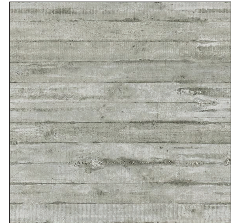
SITE FORMED CONCRETE AT LANDSCAPE WALLS
