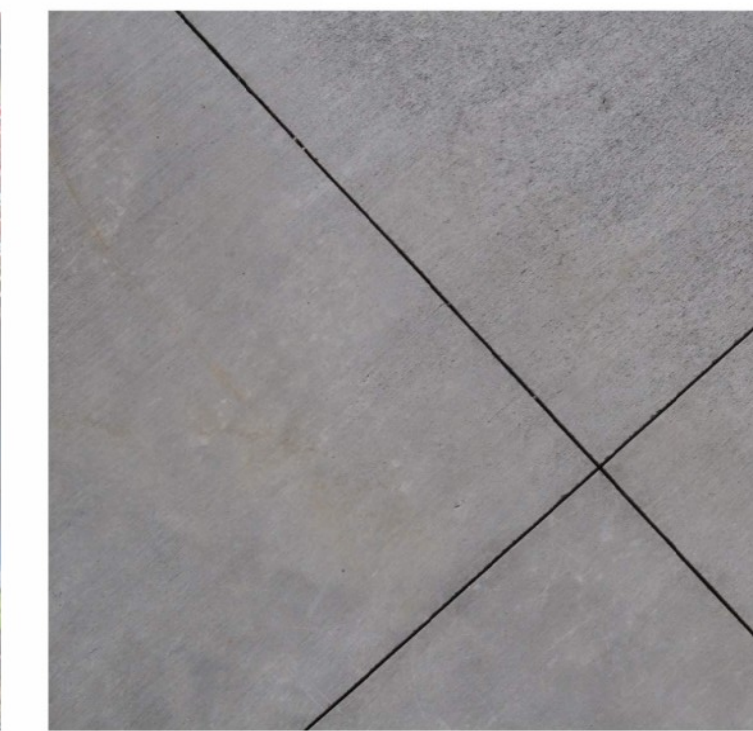
CONCRETE, BROOM FINISH, SAWCUT JOINTS
