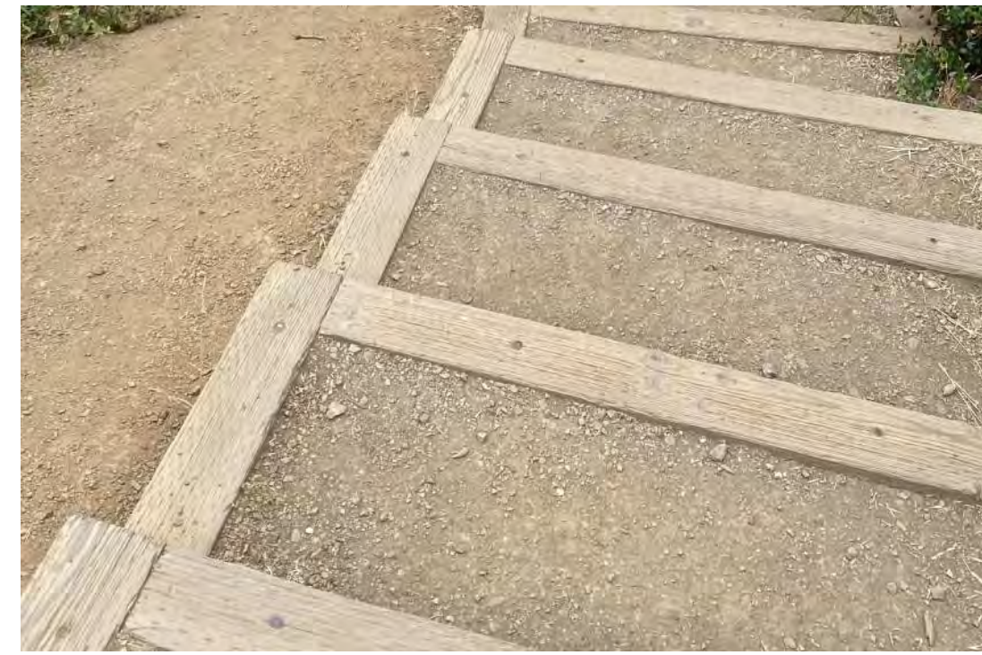
1.30 STABILIZED FINES & STAIRS
