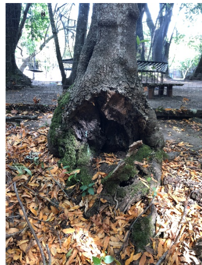
Photo 1 – California bay #46 with cavity and significant decay at root collar. Trees with destabilizing defects to this degree should be removed before the demo stage of the project begins.
