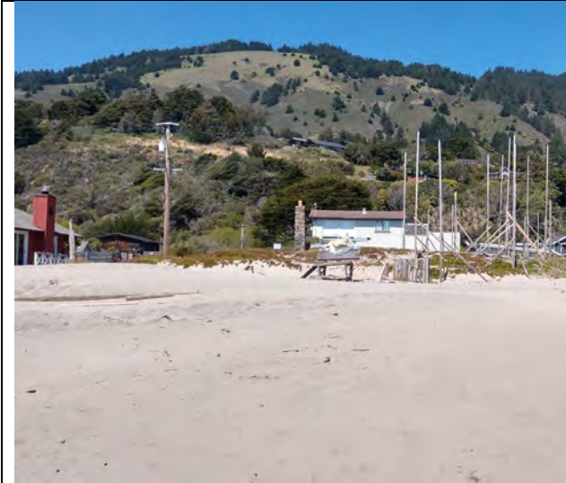
View 3: View of the Project site looking northeast prior to 2022-2033 winter season.
