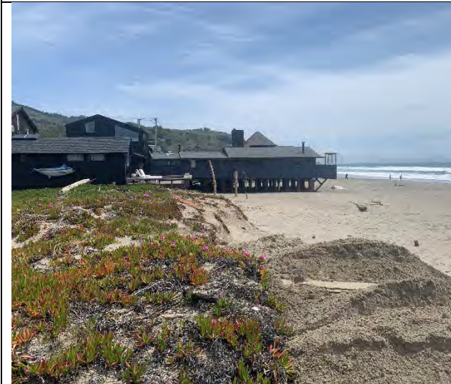
View 2: View of the Project site looking southeast from Upton Beach, April 18, 2023.
