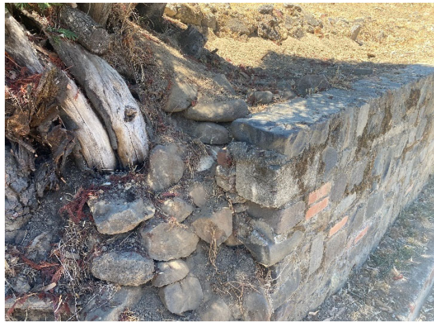
Figure 6 - Typical stacked/grouted rock wall.
