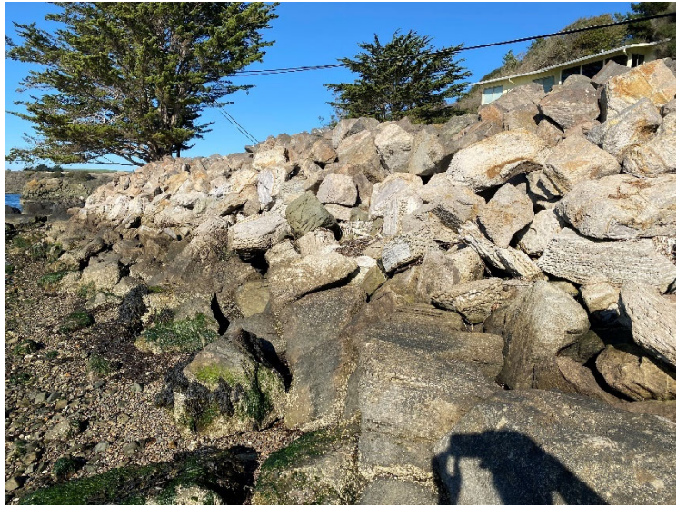
Figure 8 - Typical rock slope protection (RSP).
