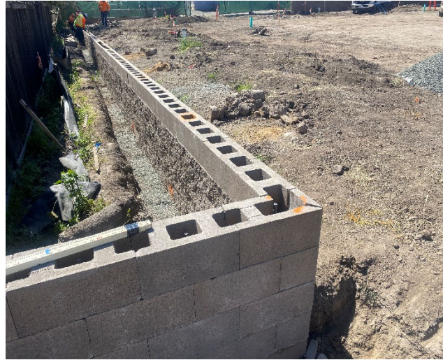
Figure 5 - Typical concrete masonry unit (CMU) wall.
