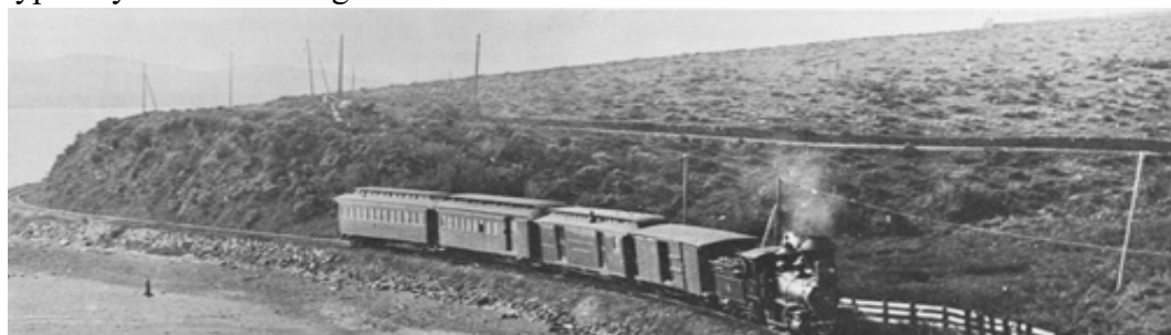
Figure 9 – Typical earth embankment. Southbound train approaching Bivalve (date unknown). Note railroad embankments were typically constructed via excavation on uphill side of tracks and fill placement on downhill side. Note RSP armoring visible on face of embankment along waterfront. (Photo credit - Tomales Bay Regional History Center).
