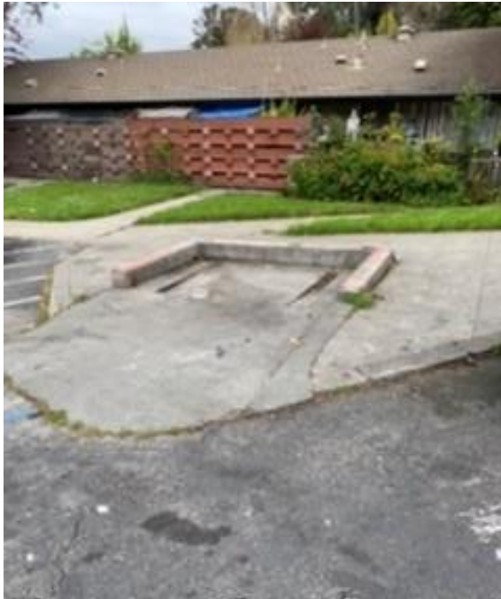
Figure 4. View of the site after one of the dumpsters was removed, near unit 23 in the parking lot off Cole Drive. Source: MHA, May 2020.
