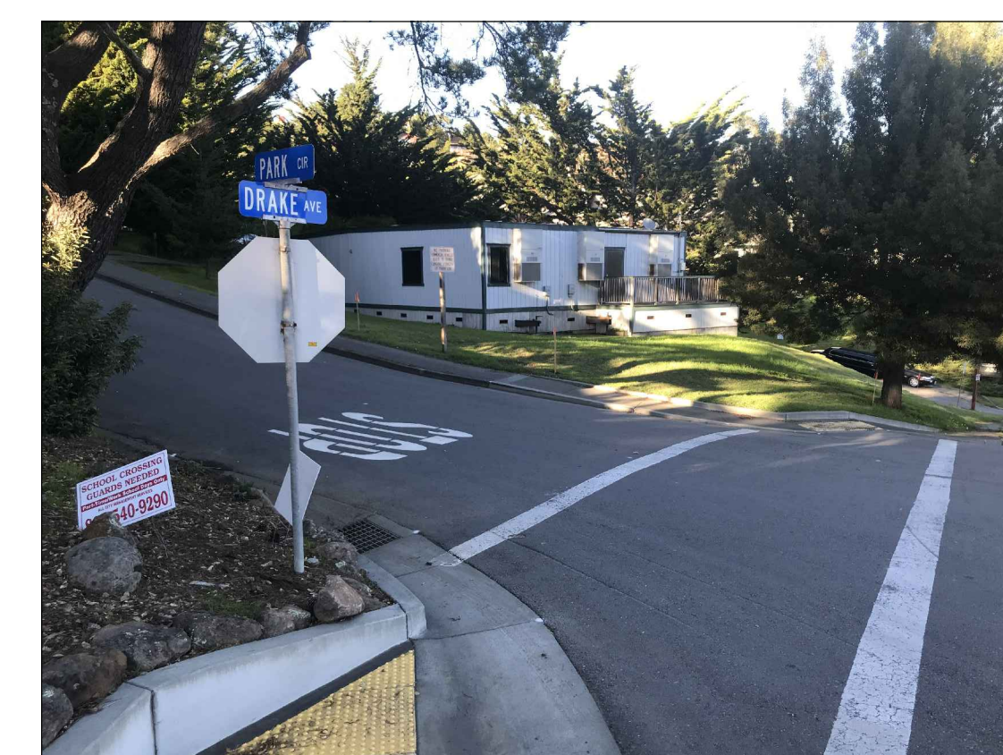
11. BUILDING LOCATED AT THE SOUTHWEST CORNER OF THE SITE WILL BE DEMOLISHED.
