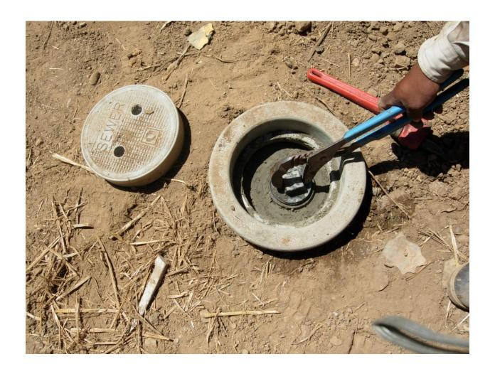
There is a difference between a performance well and a monitoring port. The monitoring ports are within a leach field trench. These ports indicate how the trench is dispersing the effluent. A performance well measures the level of ground water or wastewater in or around the area of the dispersal system.
