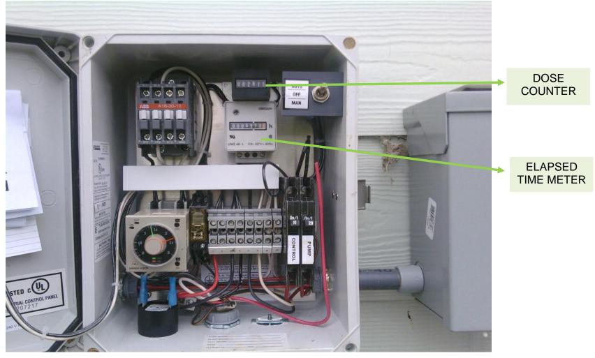
Open the control panel door. Look inside for the dose counter and elapsed time meter (ETM). If you do not have a dose counter and have an ETM (*elapsed time meter*) write in the box ETM and the readings. The dose counter tells us how many times the pump has turned on. The ETM tells how long the pump has pumped for. By reading these meters one can determine how many gallons are flowing to the septic system each day and compare it with the maximum peak flow of the system design.
