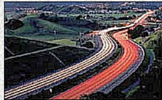
Highway 101 at the Civic Center
