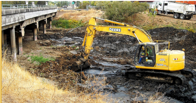
The Department of Public Works Flood Control Team conducting preventative maintenance.
