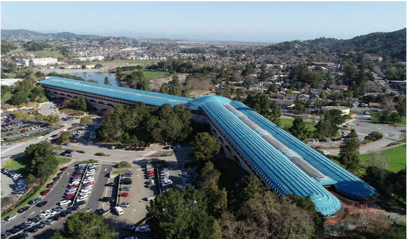
Administration Building including dome in foreground, with Hall of Justice at left rear of photo, showing new roof completed in 2020. Behind Hall of Justice is the Civic Center lagoon and park (Lagoon Park) that are part of the National Historic Landmark.
