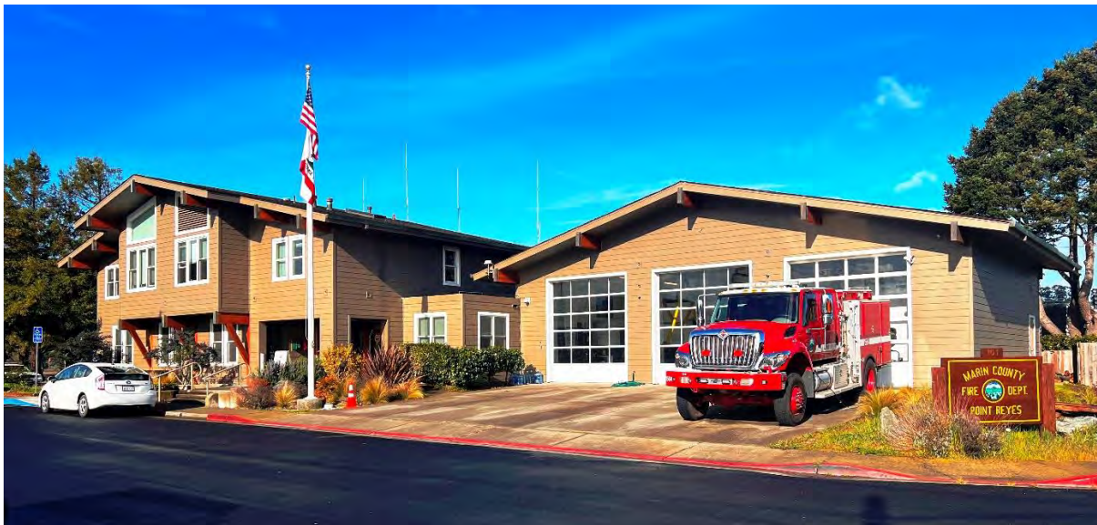
Exterior façade replacement at the Pt. Reyes Fire Station
