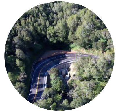
Re-pavement project by Public Works
