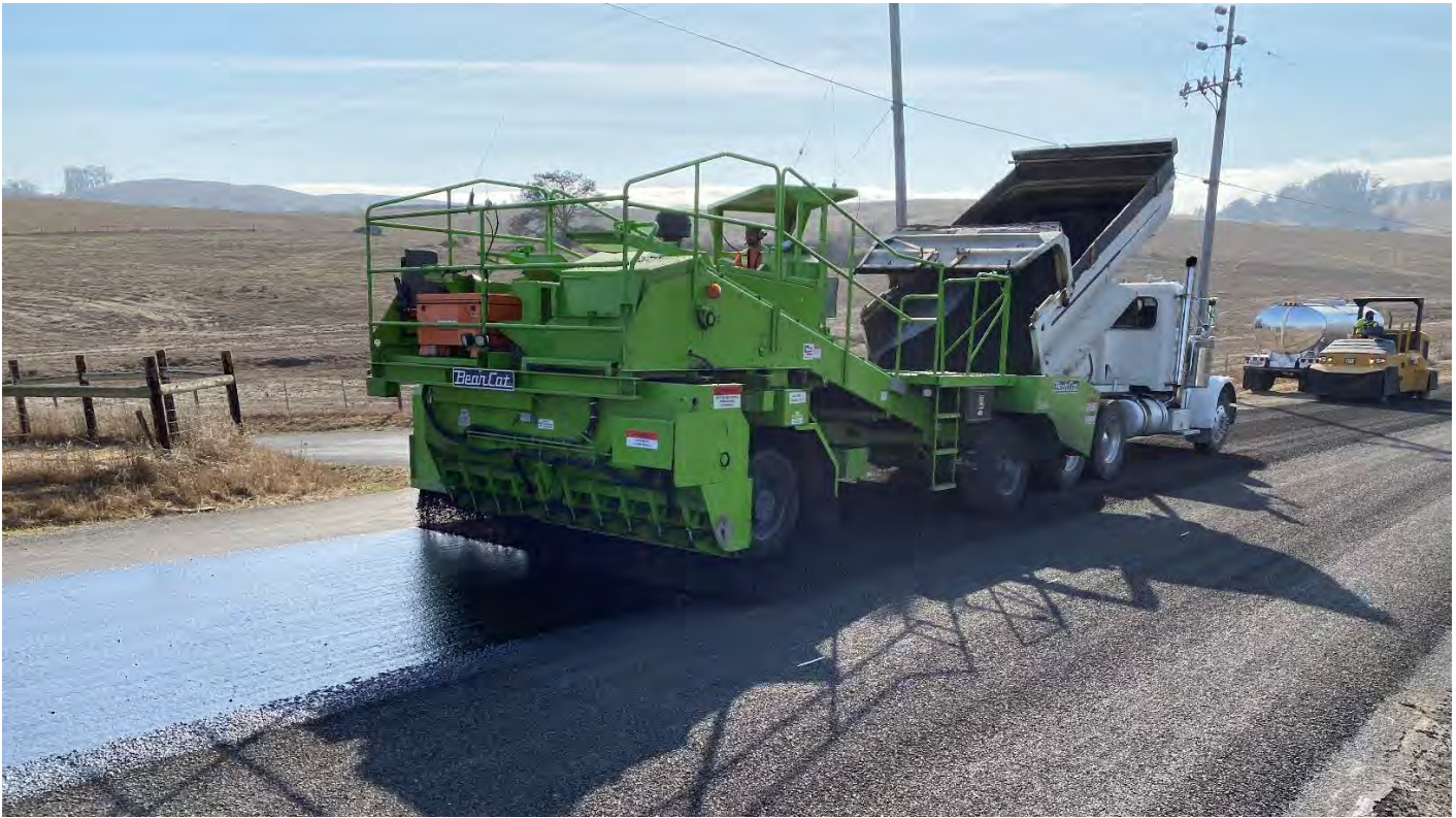
Various asphalt re-paving and sidewalk projects throughout the County.
