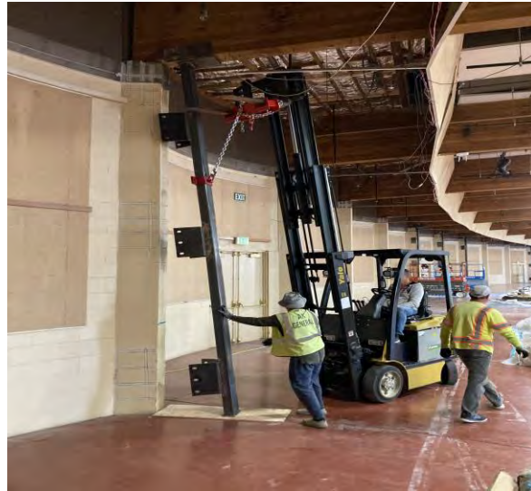
Seismic Retrofit at the Exhibit Hall
