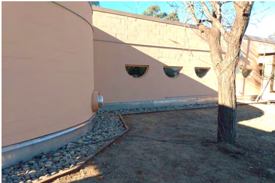
General Services Administration Building waterproofing project
