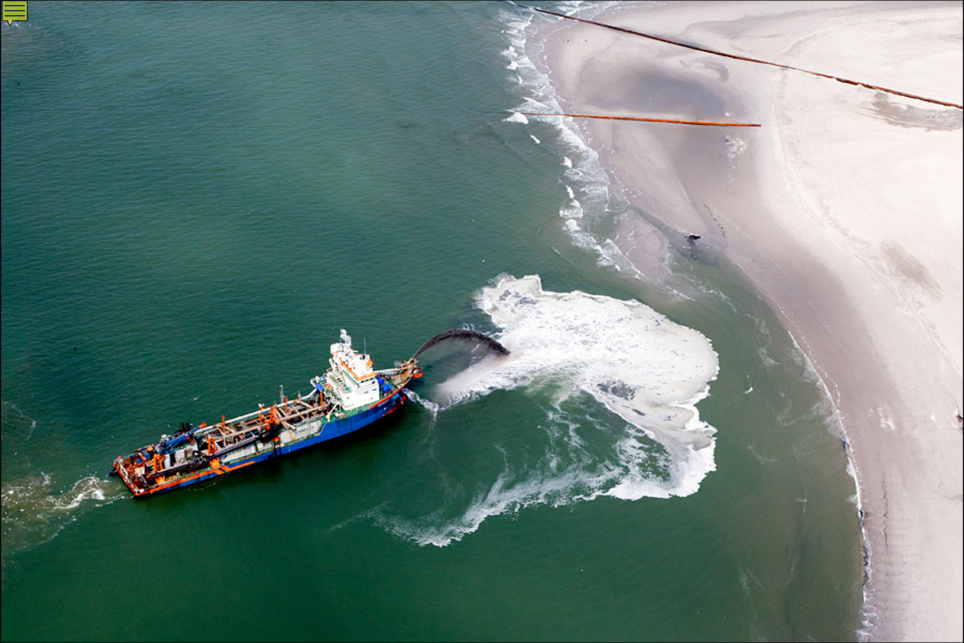
Building the “Zandmotor” using a side-caster, in addition to slurry pipes : 2011
