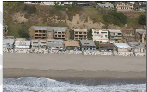
Bunker style coastal homes in Santa Cruz feature elevated ground floors that are intentionally allowed to flood
