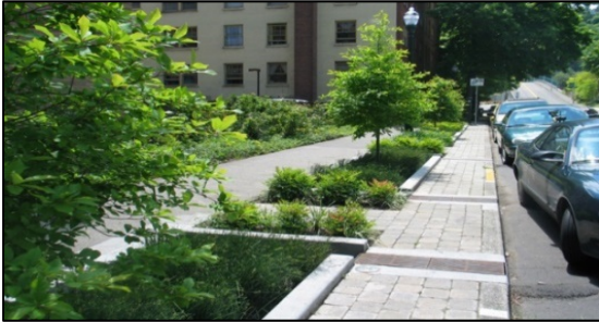
Sidewalk rain garden in San Francisco
