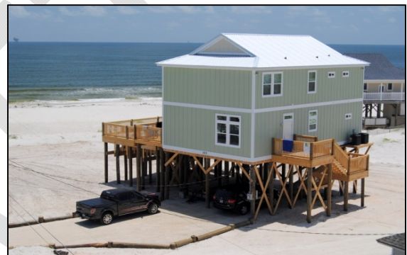
Open foundation featuring lower-level parking space
