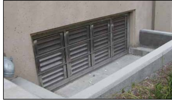
Specialized hinged vents are designed to allow water in once specific pressure loads are met
