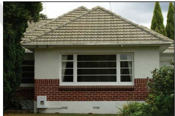
Continuous foundation wall – note new elevation walls in white
