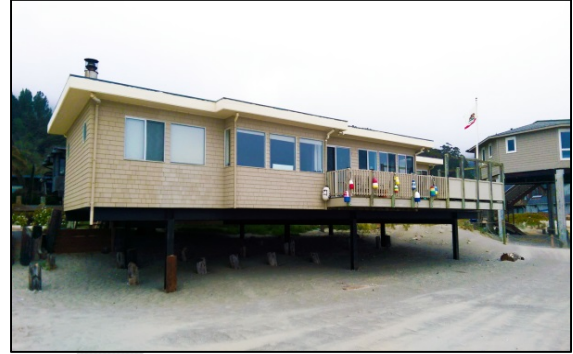
Elevated beach home with open foundation
