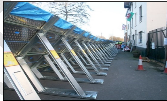
Temporary floodwall represents an alternative to sandbagging
