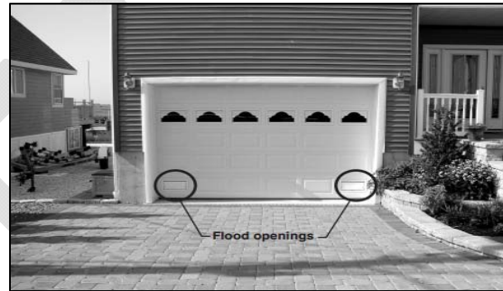
Openings incorporated into a garage door allow for entry of water
