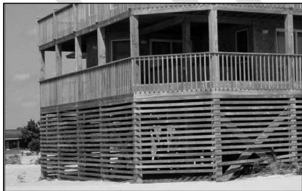
Wood slats installed over pilings to hide open foundation
