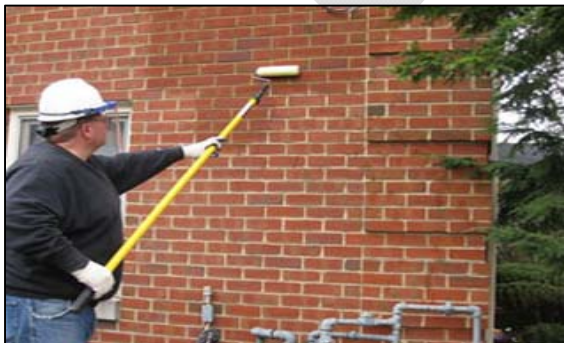
Sealant applied like paint on exterior walls
