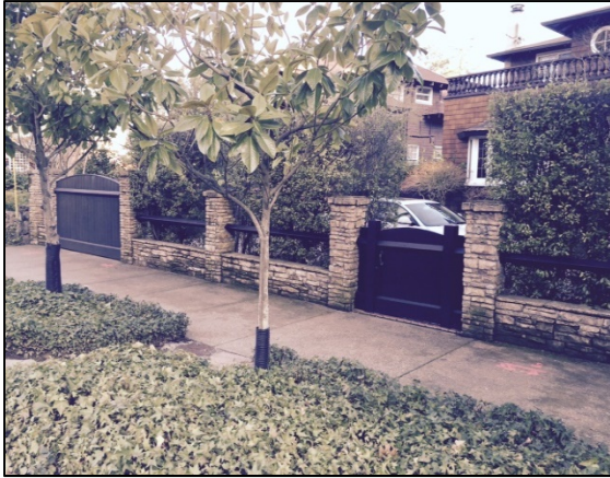
Flood wall and gate applied in a residential setting and masked with landscaping
