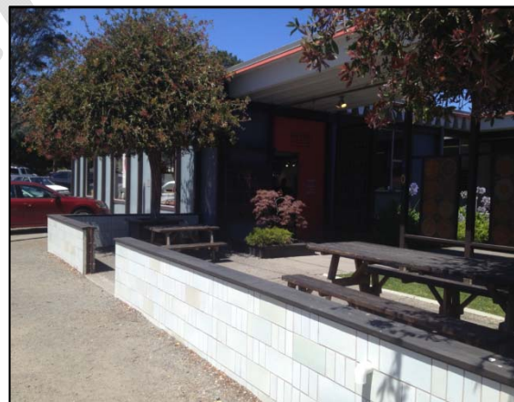
Low-tiered flood wall and gate installed at a commercial building in Marinship. Opening allows for manual insertion of a flood barrier.
