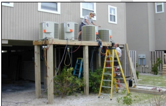
Mechanical equipment relocated to higher
