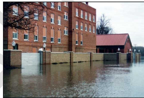
Successful application of dry floodproofing barrier in North Dakota
