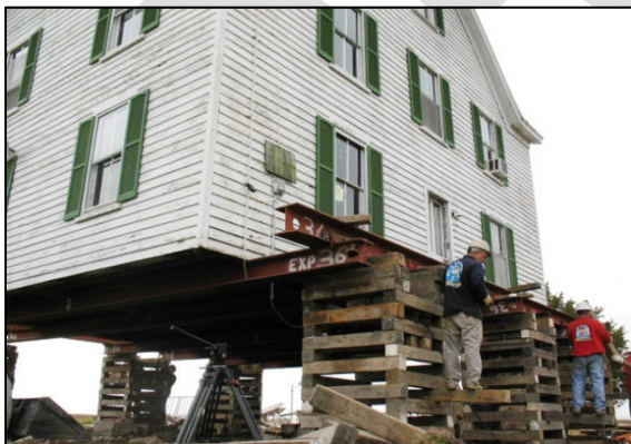
Home resting on temporary beams and foundations
