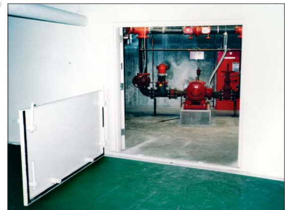
Hinged flood shield designed to protect utility systems at a moment's notice
