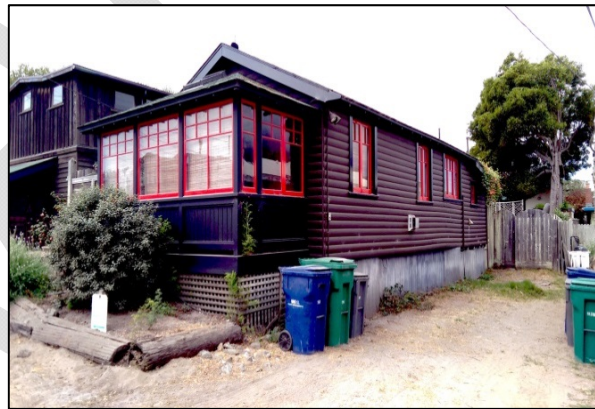
Coastal home with slight raise, masked with landscaping and wood-lattice
