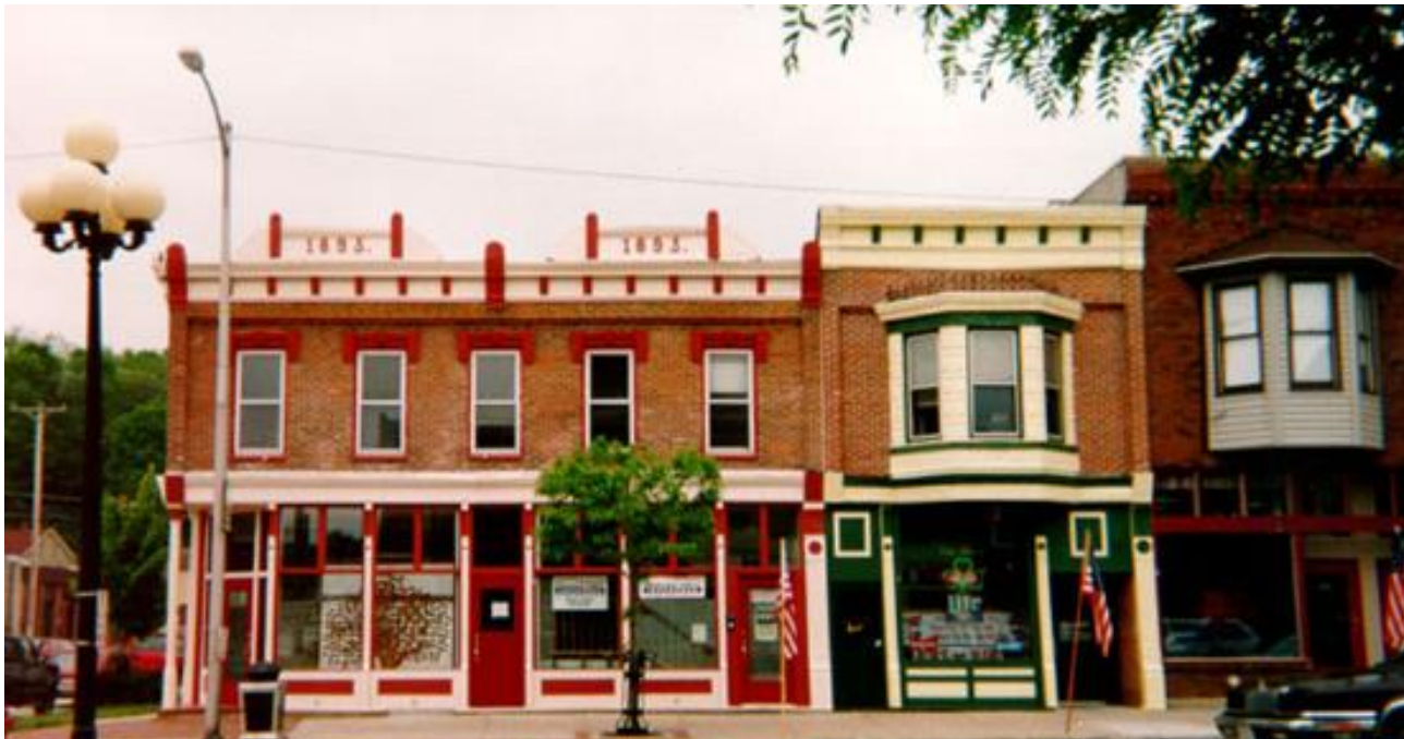
Retrofitting buildings in Darlington, Wisconsin
