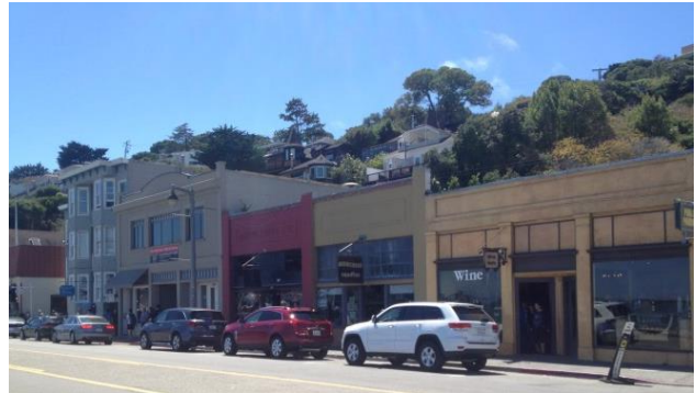
In the long-term flooding could impact Bridgeway and historic buildings lining its west side. Credit: Marin County CDA
