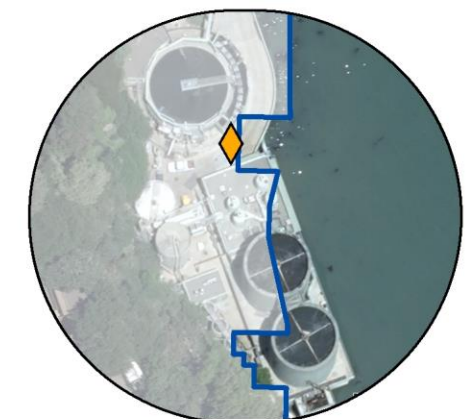
4: Sausalito Marin City Wastewater Treatment Plant
