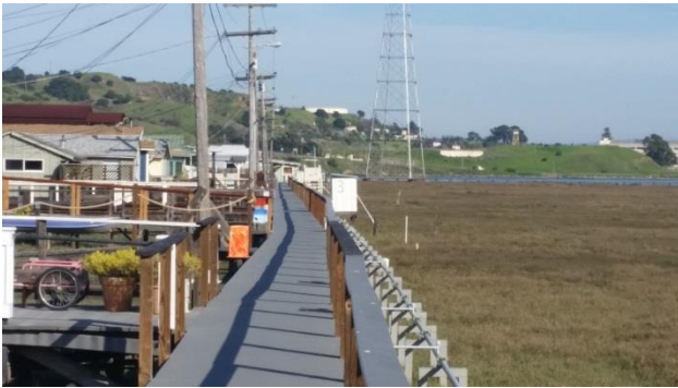
Greenbrae Boardwalk. April 2016. Credit: BYB Consulting LLC
