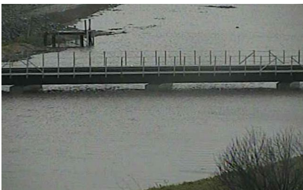
SMART Bridge, Novato. Credit: Marin County DPW
