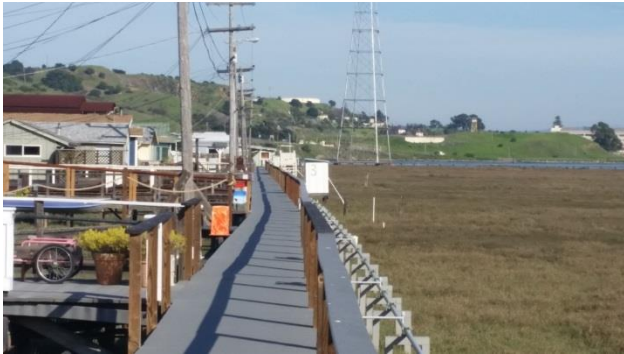
Greenbrae Boardwalk. April, 2016. Credit: BVB Consulting LLC
