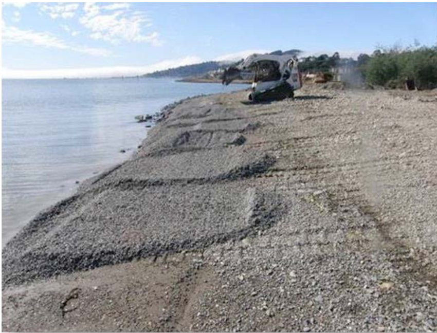
Figure 2: Placing gravel along Aramburu Island shoreline.
