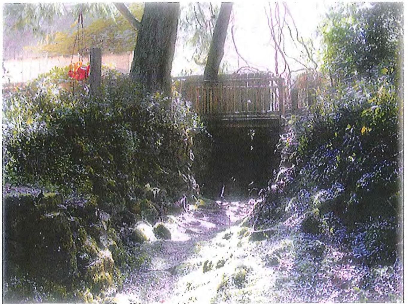
Dry ephemeral stream within 10 feet of house.
