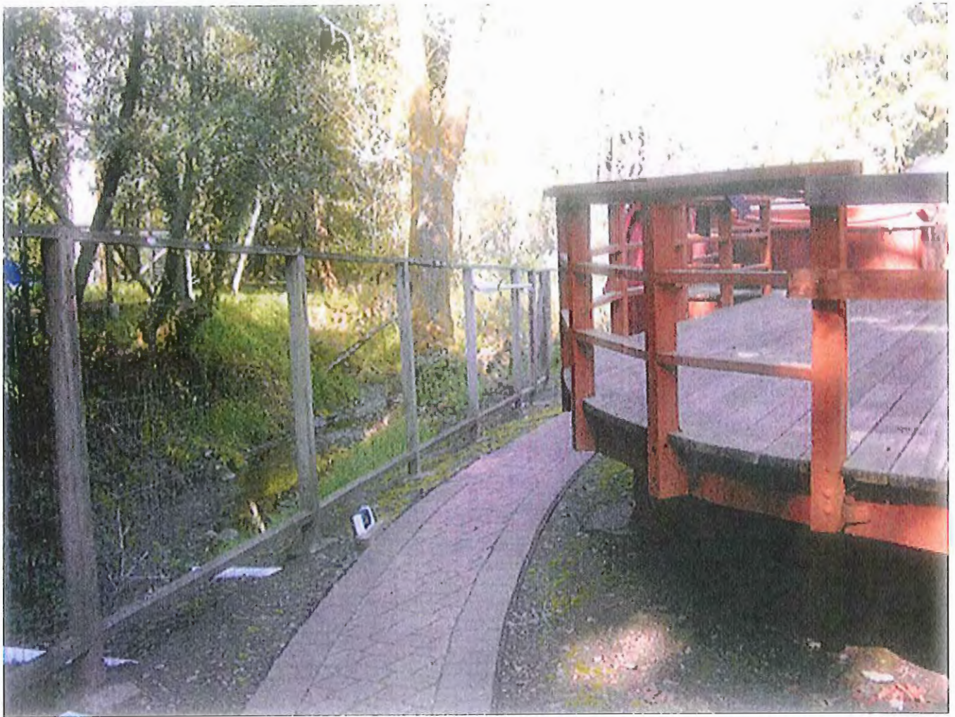
Seasonal Stream within 10 feet of Deck and fence.
