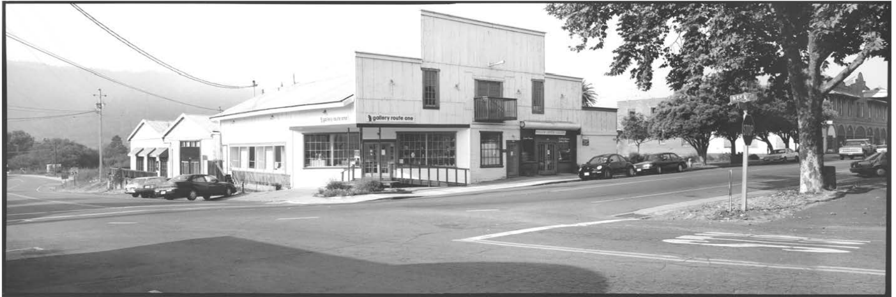
Corner of First and Main – Cheda Building
