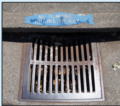
Storm drain on Vendola Drive
