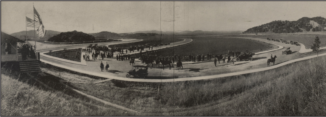
McMahon's development scheme for Santa Venetia involved raising the marsh by 6-8 feet from 1908-1914
