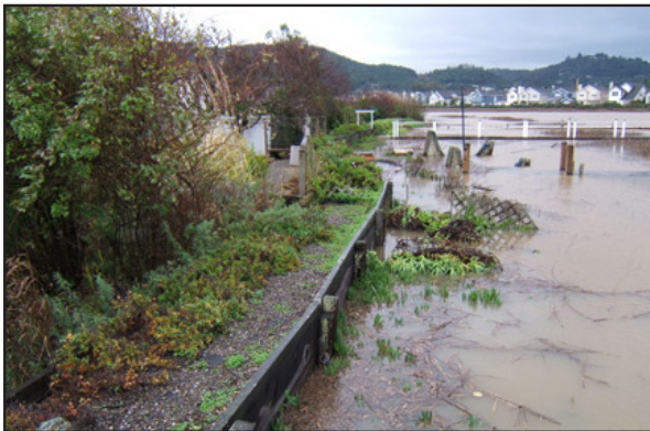
High tides approach the top of the existing levee in 2006
